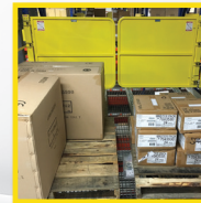
Pallet Rack Safety Gate
